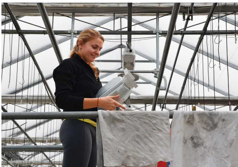
Figures 4a & 4b. A high-pressure sodium reflector has been removed from the fixture and is ready to be cleaned.
