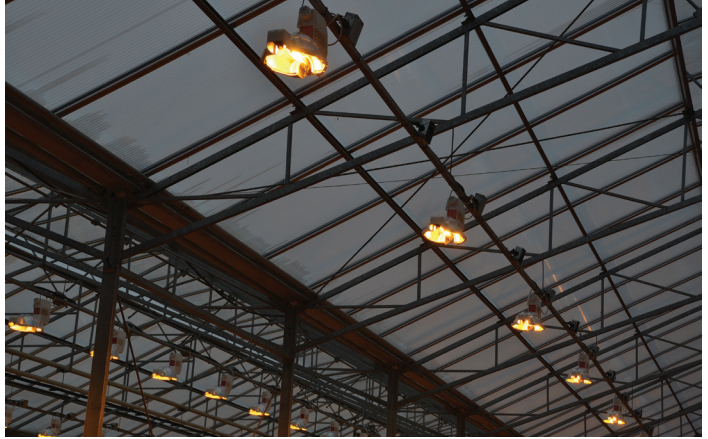
Figure 1. Northern greenhouse operation using supplemental lighting from high-pressure sodium lamps to provide 150 \mu\text{mol}\cdot\text{m}^{-2}\cdot\text{s}^{-1} to their cucumber crop.
