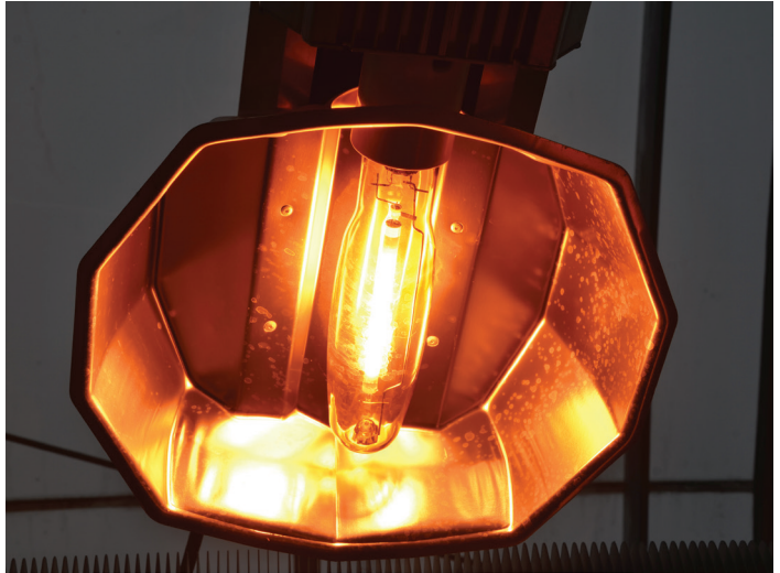
Figure 3. Reflector and bulbs with dust, finger prints and water spots
